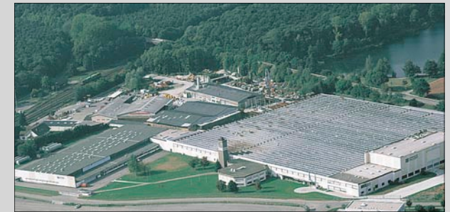
Main facility in Malterdingen
